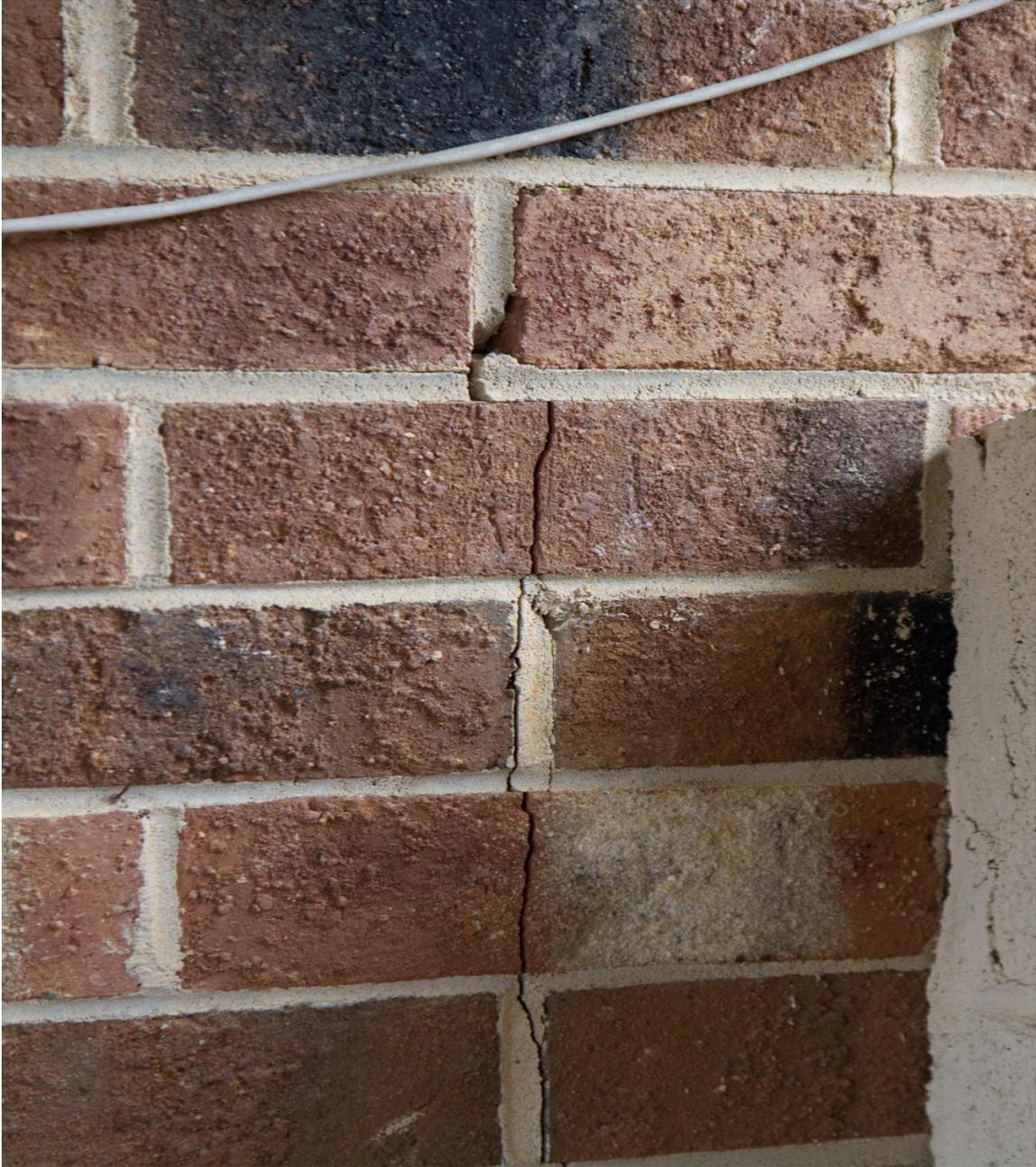
Small crack in foundation under front porch. There is very little separation of shifting visible at this time but this should be monitored.
